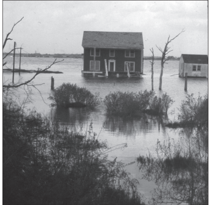
Figure 7. Abandoned house in the Brownswood subdivision in Baytown, Texas, in the Houston metropolitan region. Pumping of groundwater caused land to subside below Galveston Bay. Photograph by Charles W. Kreitler, 1975.
