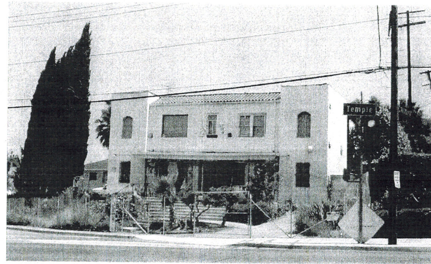
Derelict apartment building on Temple Ave..
